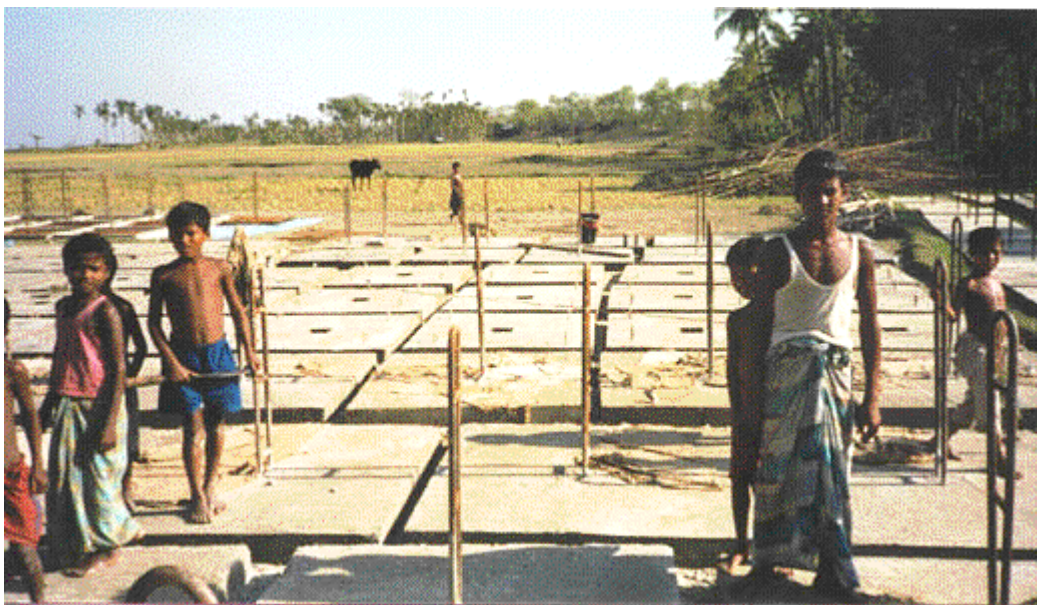
Figure 15: Shows the reinforced concrete plates that DEFT are building.
